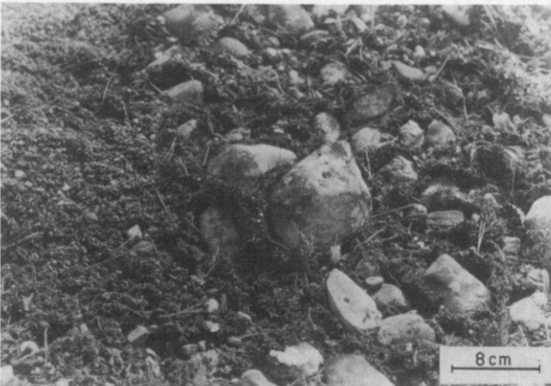
Photo 3: Gaps around stones.
